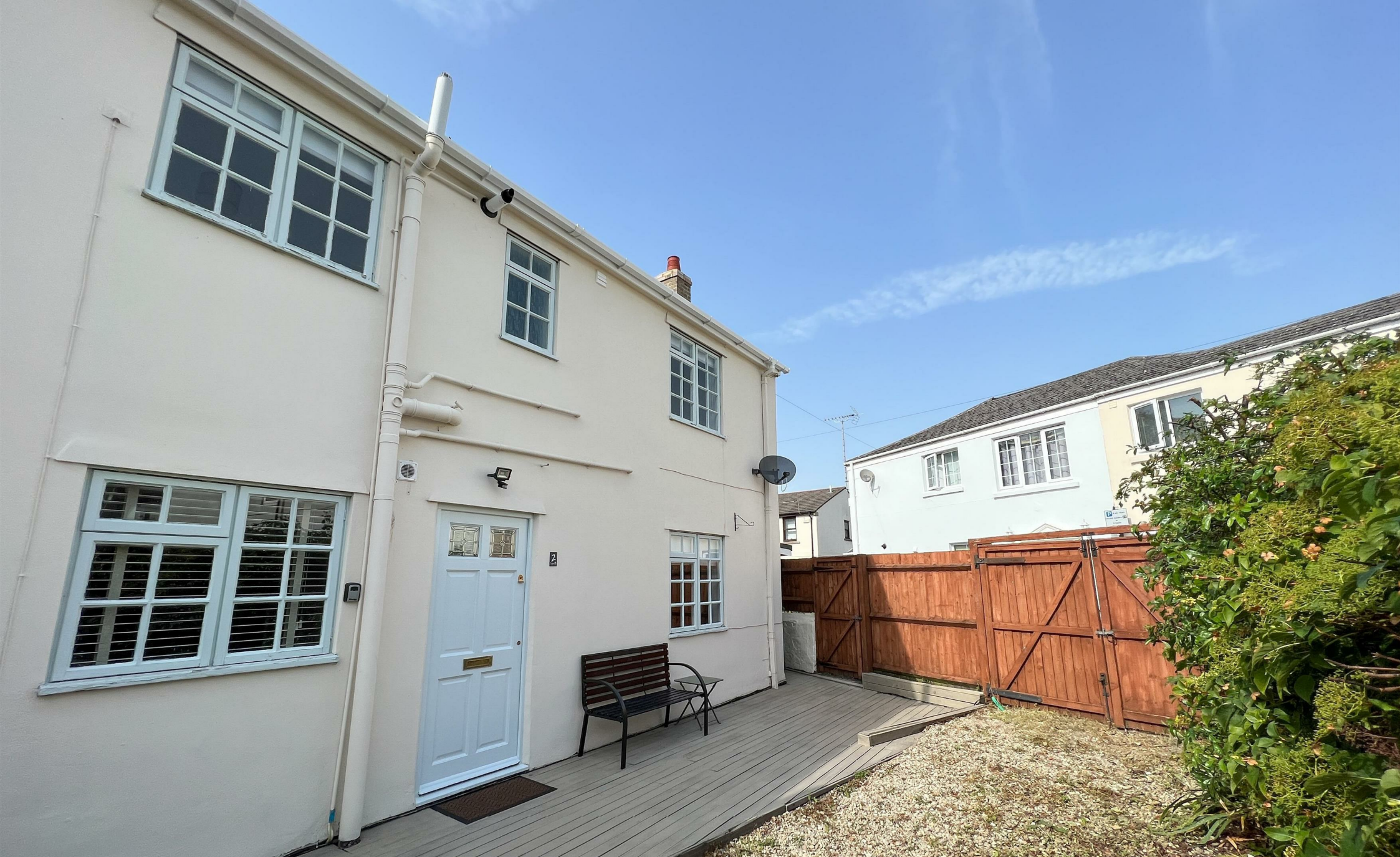
2 Providence Cottage, Andover Road, Cheltenham, Gloucestershire, GL50 2EF
