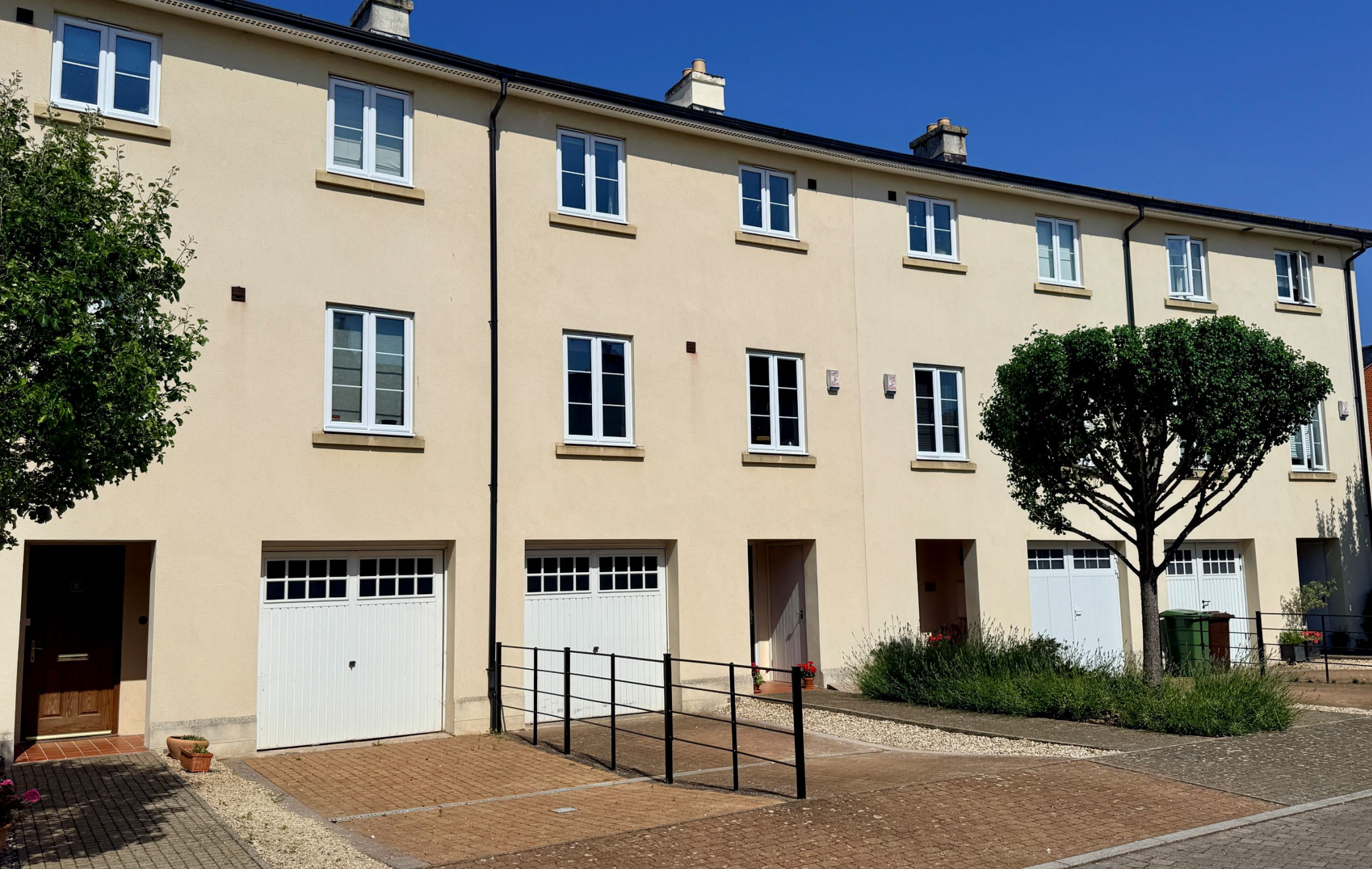
6 Arthur Bliss Gardens, The Park, Cheltenham Gloucestershire GL50 2LN
